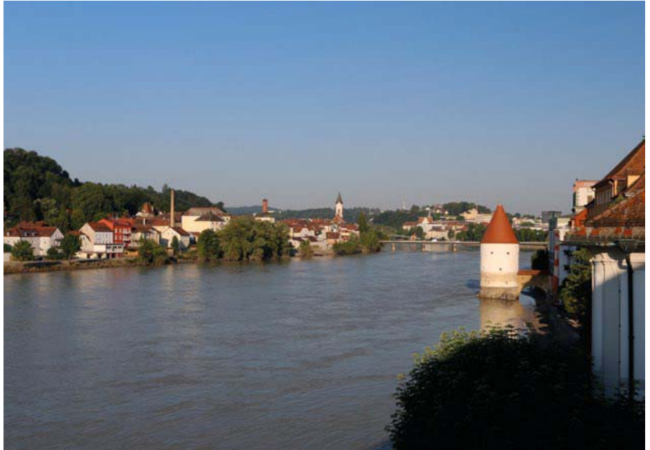
Damage from the June 2013 flood along the Inn river, shown at a stage when it still exceeded flood warning levels. (Photo: Michael Szönyi)
