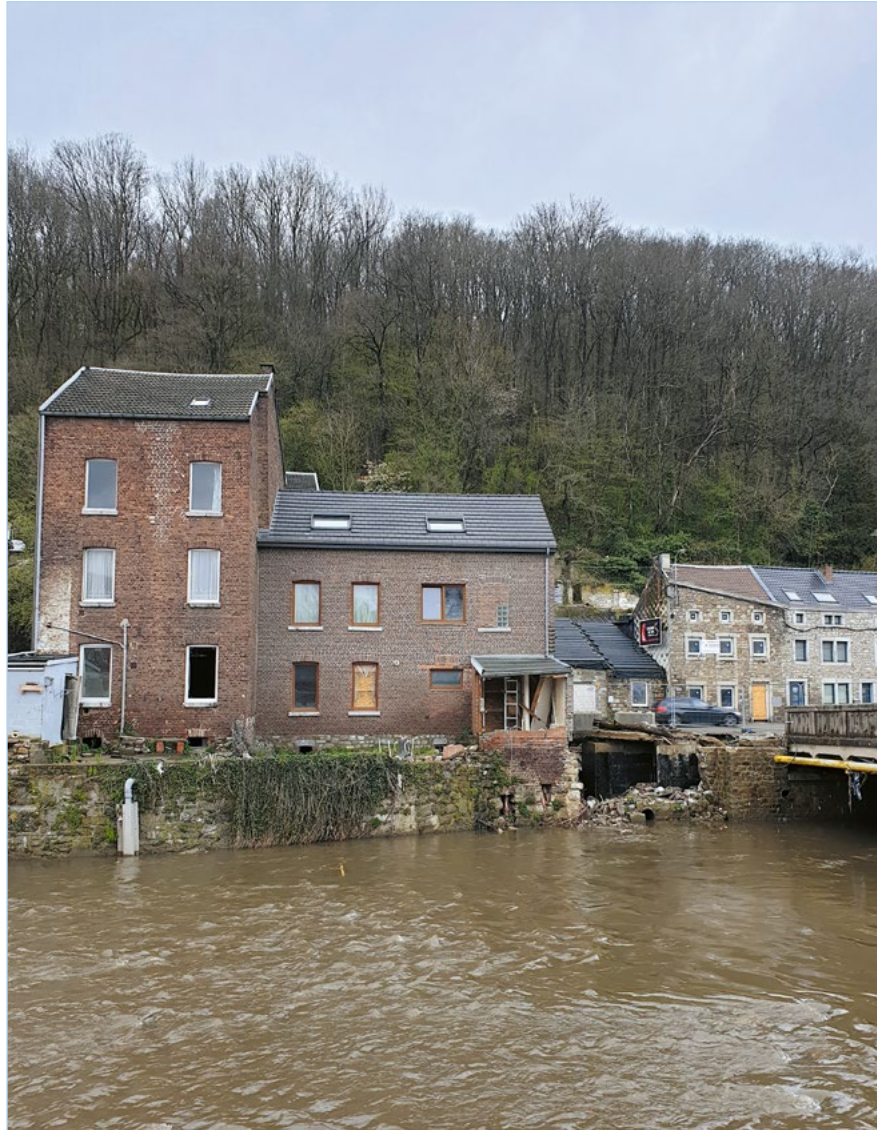
Photo: Many houses nestled along the Vesdre in Verviers, Belgium, were destroyed during the summer 2021 floods. Teresa Deubelli, IIASA.
