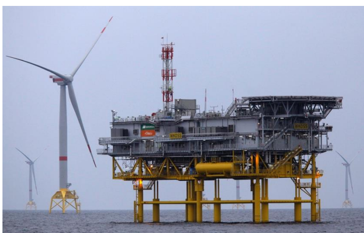
Iberdrola's offshore windfarm 'Wikinger' in the Baltic Sea. Source: Iberdrola, June 2018
